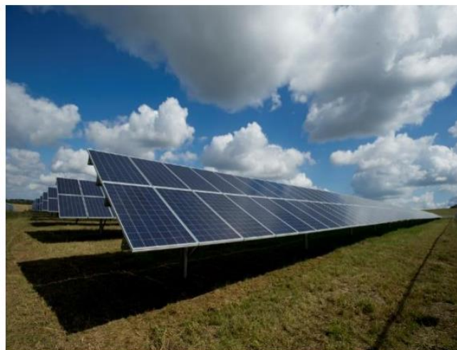
Figure 2 - Example of fixed tilt panel orientation
